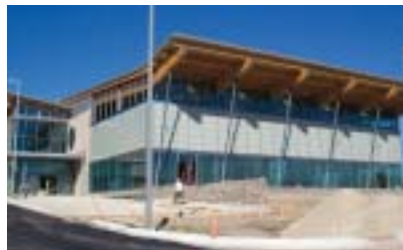
New and bigger facilities, like the Angus Glen Pool in Markham shown here, require a diligent risk management strategy to maintain safety standards.
